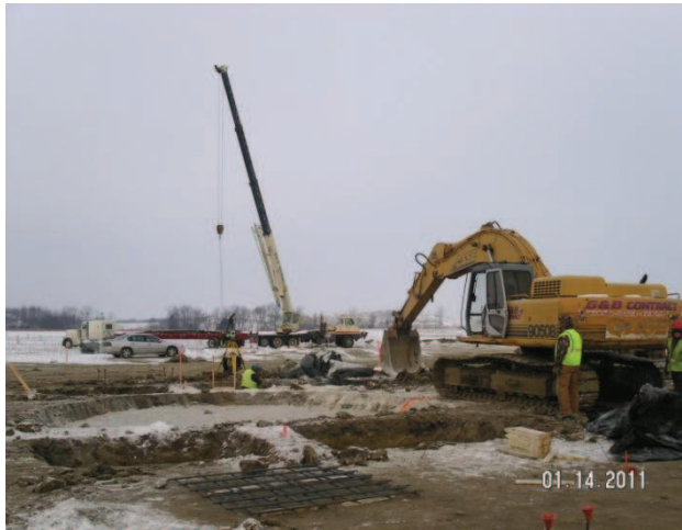
Figure 1 Description: Building 2: J&J Steel unloading rebar. Scurto Concrete forming footings. 01/14/2011
